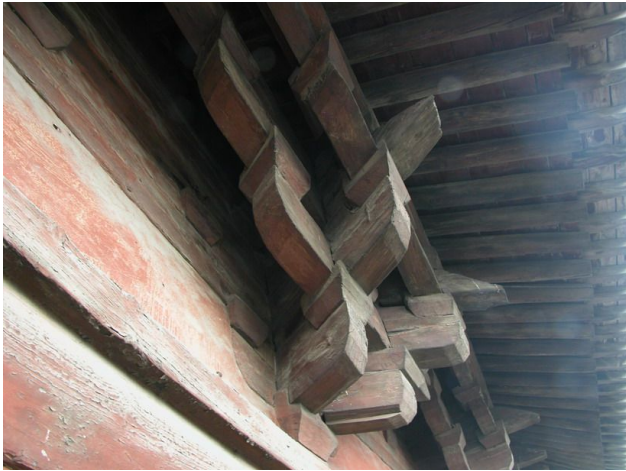
Fig.17 Shanhua Temple—The Inclined Dougong of Samantabhadra Pavilion. Copyright 2011 JI Jianle, all rights reserved used by permission
