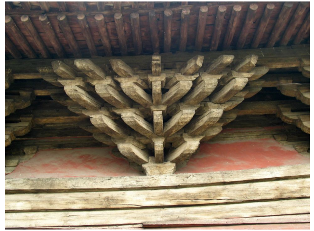
Fig.14 Shanhua Temple—The Inclined Dougong of Sanshengdian. Copyright 2011 JI Jianle, all rights reserved used by permission
