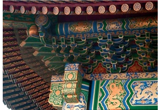
Fig.30 ougong of Qing's architecture. Copyright 2011 JI Jianle, all rights reserved used by permission
