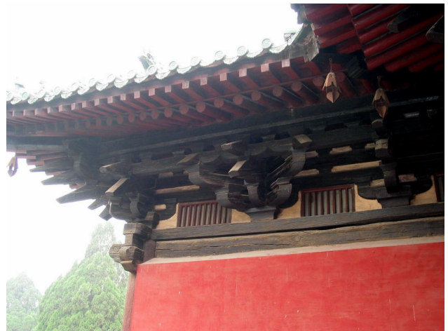
Fig.24 Dougong of Song's architecture. Copyright 2011 JI Jianle, all rights reserved used by permission
