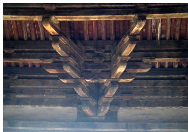
Fig.19 Shanhua Temple—Inside of the Inclined Dougong of the Main Hall. Copyright 2011 JI Jianle, all rights reserved used by permission
