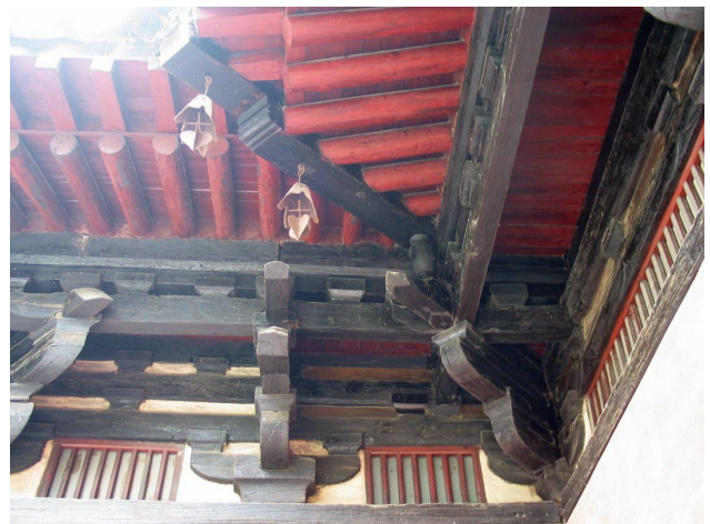
Fig.25 Dougong of Song's architecture. Copyright 2011 JI Jianle, all rights reserved used by permission
