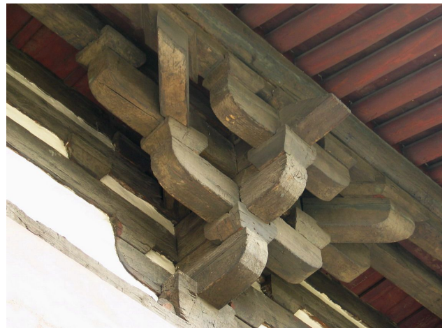
Fig.20 Shanhua Temple—Outside of the Inclined Dougong of the Main Hall. Copyright 2011 JI Jianle, all rights reserved used by permission
