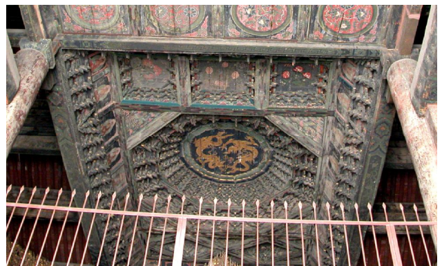
Fig.21 Shanhua Temple—The special sunk panel of the Main Hall. Copyright 2011 JI Jianle, all rights reserved used by permission
