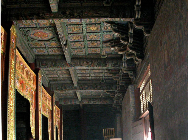
Fig.7 Northern Huayan Temple—Dougong and Ceiling of the Main Hall. Copyright 2011 JI Jianle, all rights reserved used by permission
