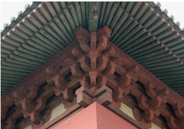
Fig.8 Northern Huayan Temple—Dougong of the Main Hall. Copyright 2011 JI Jianle, all rights reserved used by permission
