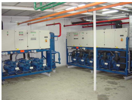
Figure 13 – Refrigeration machine room
