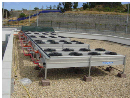
Figure 14 – Condensers located in roof
