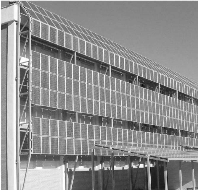
Fig. 7. Photography of 'Façade' system
