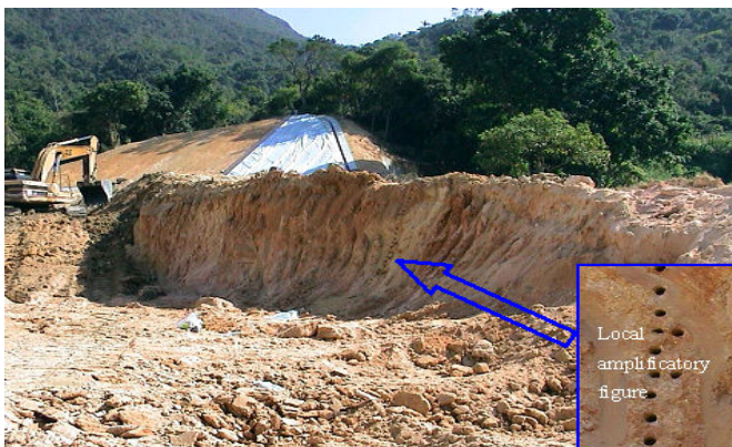
Fig. 3 Photo of the site and section of samples from MA ON SAN.
