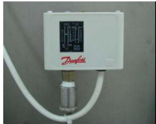
Fig. 9 pressure sensor
