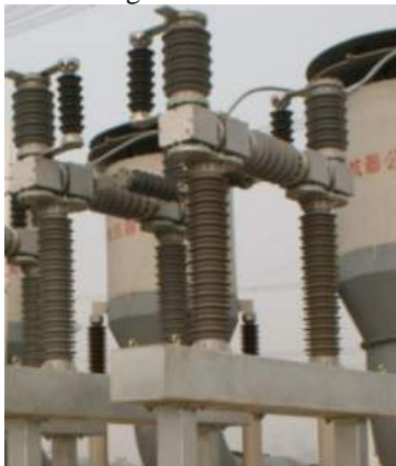
Fig. 13. Module of VCB with triple interrupters
