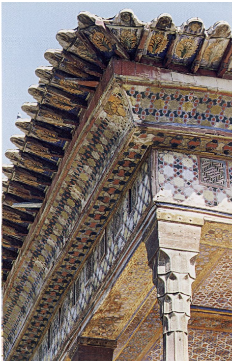
Fig. 9 Wooden roof and column of Chehelsotun Palace
