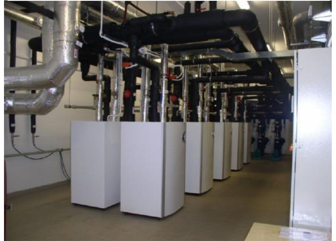
Fig. 13a BRP heat pumps located at junction wells of the Nova aula building [7]
