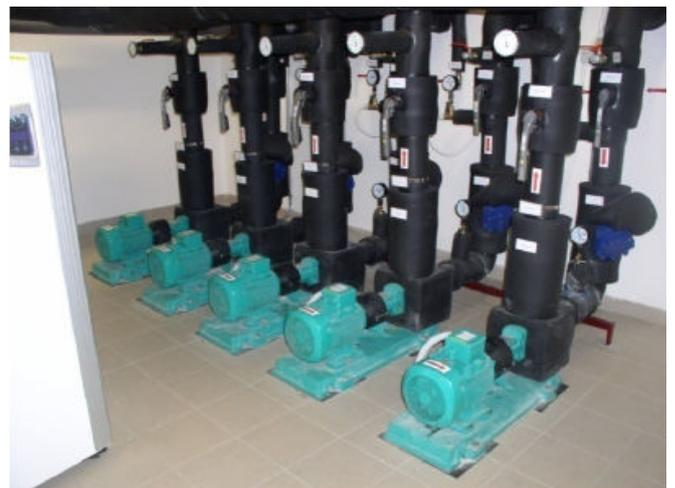
Fig. 13b five circulation pumps, used for primary circuit of the BRP heat pumps [7]
