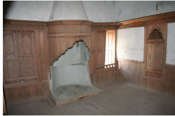
Photo. 1- Interior view of a room.
