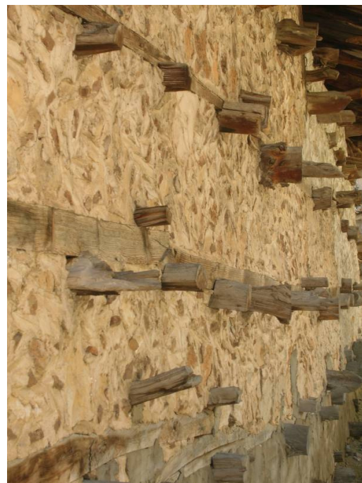
Photo. 3- Detail of construction
