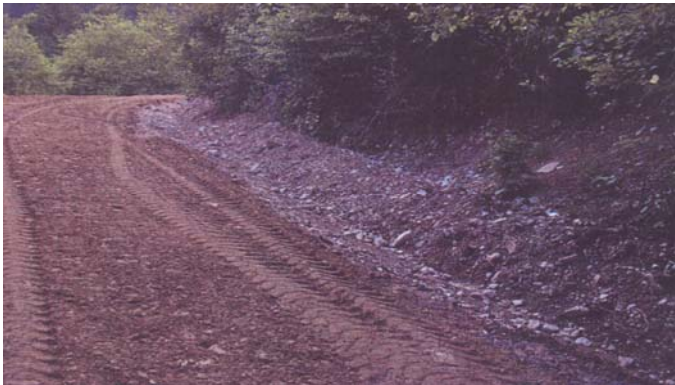
Fig. 8 – Finished platform and ditches
