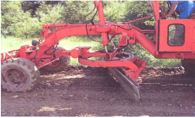
Fig. 7 – Finishing works with grader
