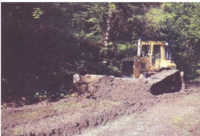
Fig. 5 – Embankment realization with bulldozer
