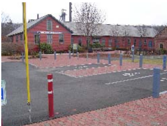
Fig. 3. The Great Falls Discovery Center is located in the former Montague Paper Company facility.
