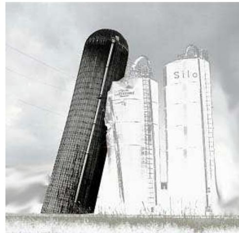
Fig. 2. Collapse of a silo due to a poor design.
