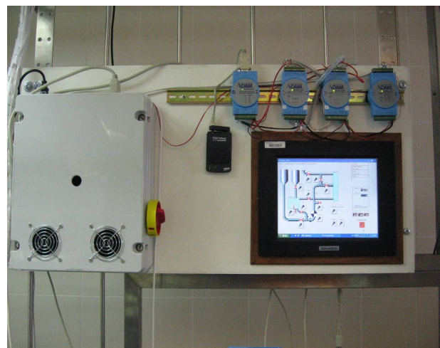
Fig 4 control board with panel PC, ADAM modules and converter box.
