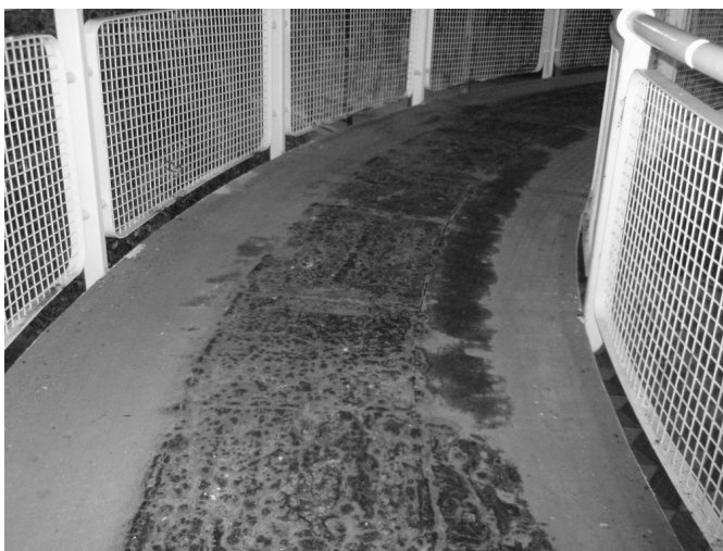
Fig. 3 Actual condition of the transversal section of the footbridge.
