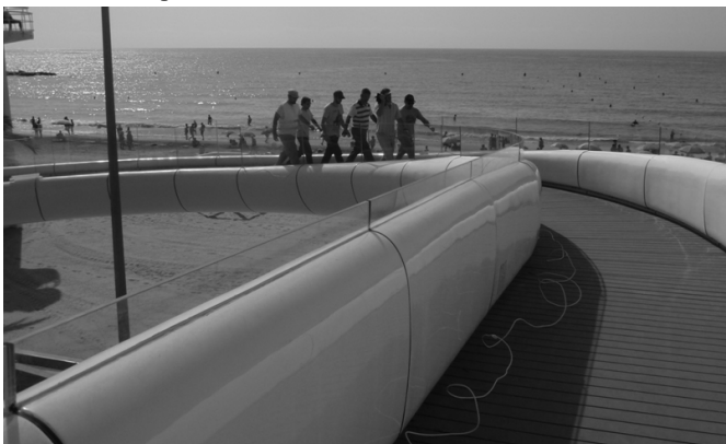
Fig. 16 Group of 6 pedestrians walking on the footbridge
