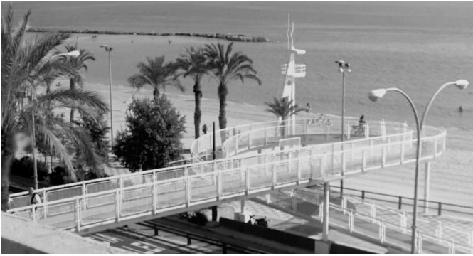
Fig. 2 Pedestrian bridge. Postiguet beach, Alicante, Spain.
