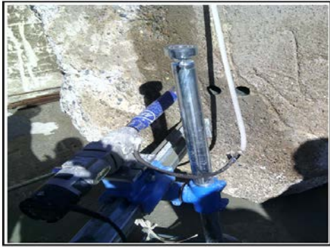
Fig. 3 GCB coring in concrete.
