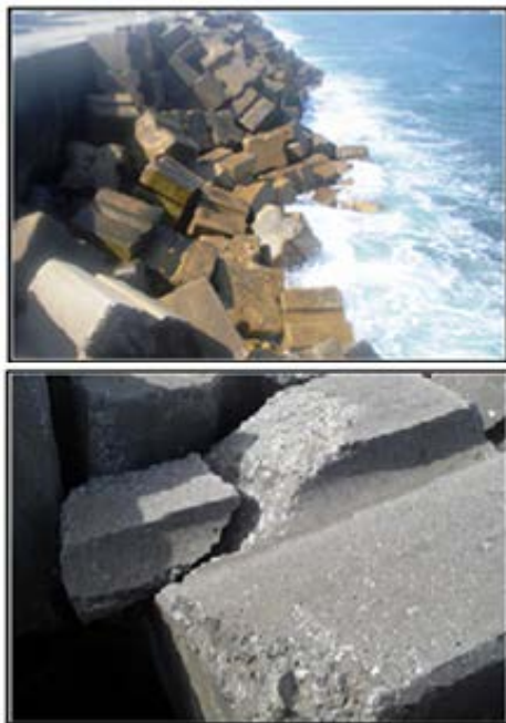
Fig. 1 shelling GCB at the coronation of the pier North West of the port DjenDjen.
