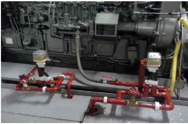
Fig. 9 Erection of flow meter (after)
