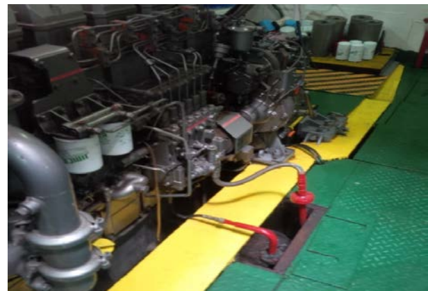
Fig. 8 Erection of flow meter (before)
