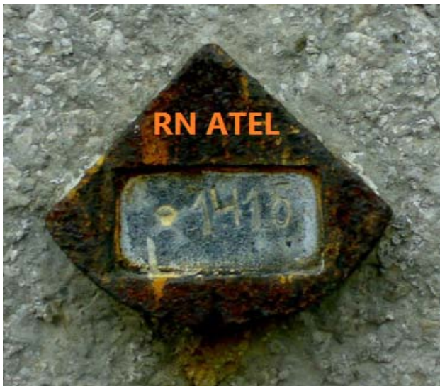
Fig. 9. A benchmark placed in a railway station
